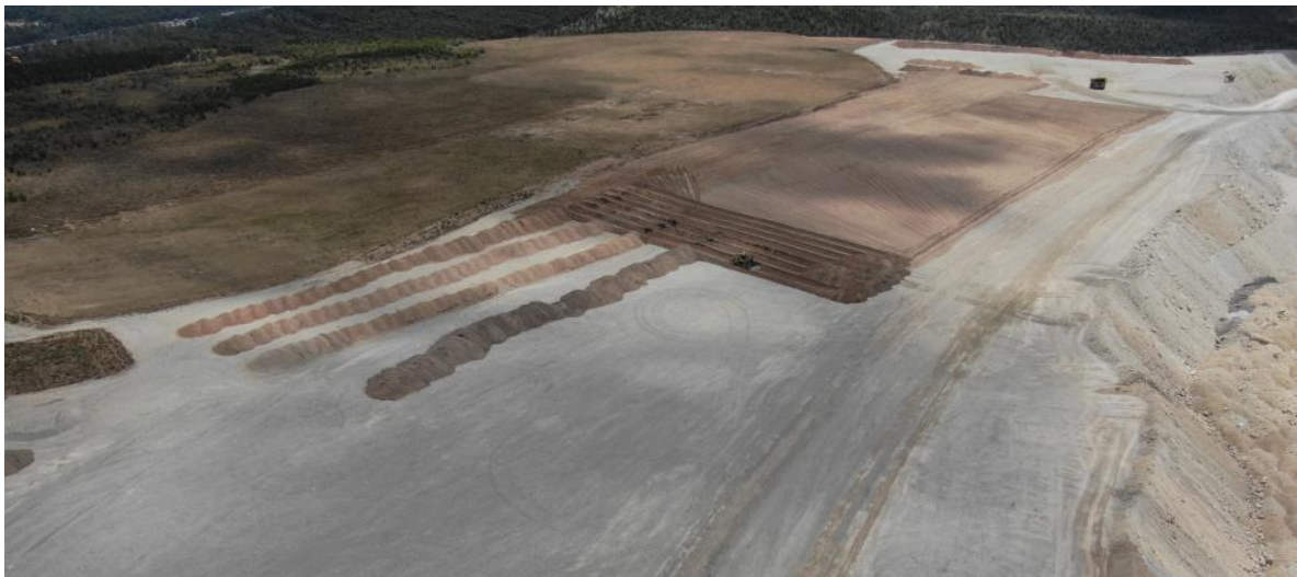
Figure 3 North Rehab – Subsoil being pushed out over recently landformed area (January 2025).
